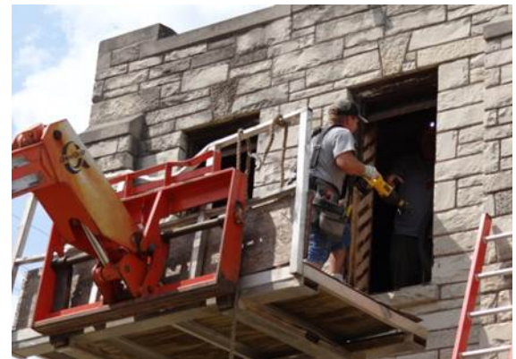
Work on the Louver's at Zion
